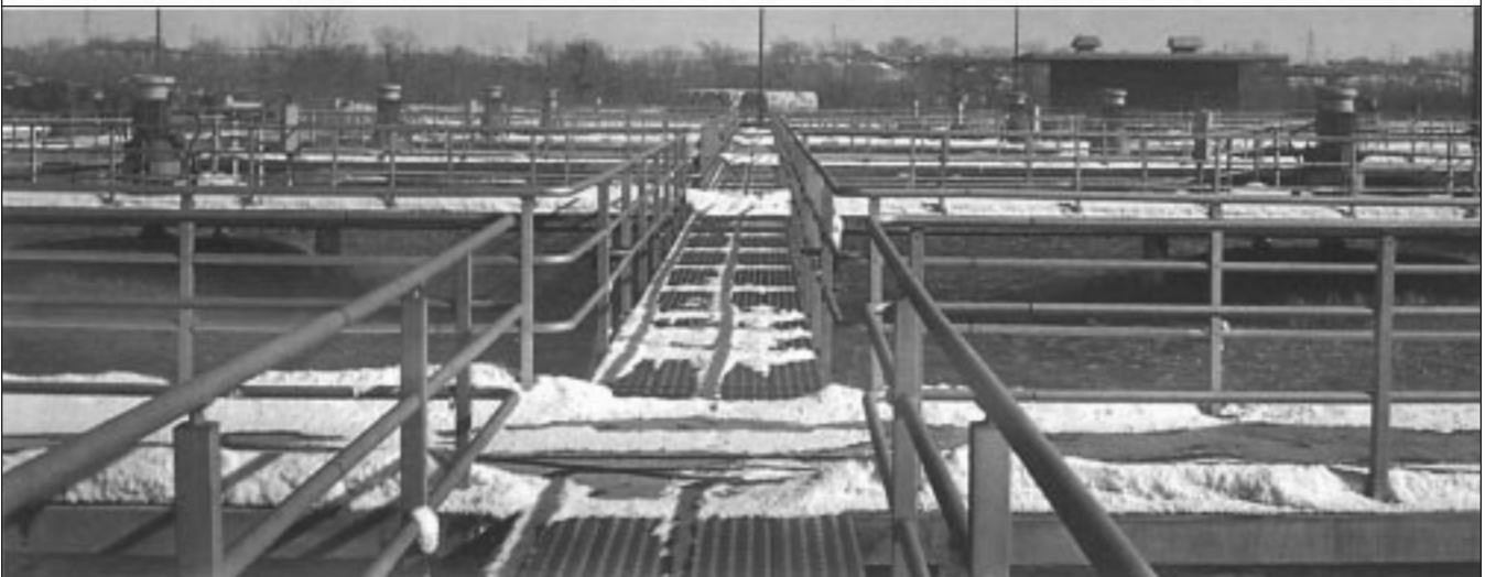
Bonny Brook Sewage Treatment Plant, Calgary, Alberta
